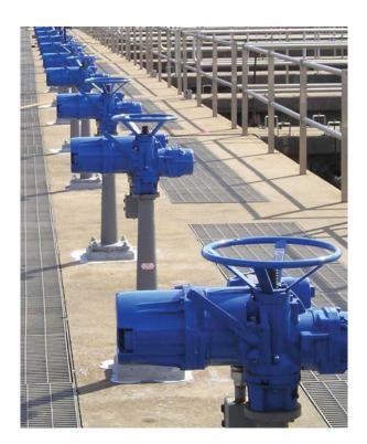
first unit was shipped in 1997. It was the first non-intrusive actuator to use rolled worms and electronic controls designed and produced using surface mount technology. A true globally certified device, MX meets all pertinent European Directives including ATEX, EMC, Machinery and Noise and displays the CE mark associated with such compliance.
